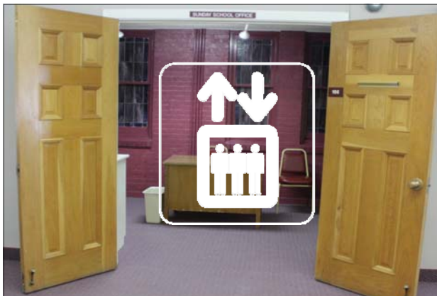
Current Sunday School office on 1st floor is the site for three-floor elevator in main building. Storage rooms on 2nd floor and basement would be converted to the elevator.
